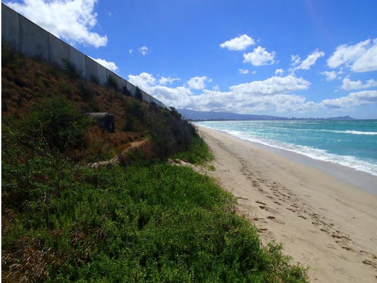
Figure 3. The ocean side of the long-distance ranges consists of tall earthen berms with concrete barriers on top.
