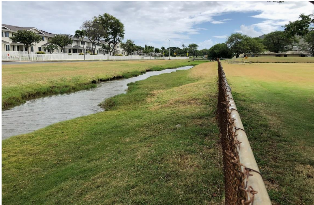
Figure 6. Mokapu Central Drainage Channel.
