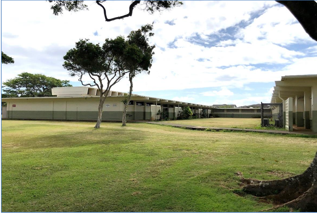
Figure 5 – Mōkapu Elementary Playground, showing mowed grass and school buildings.
