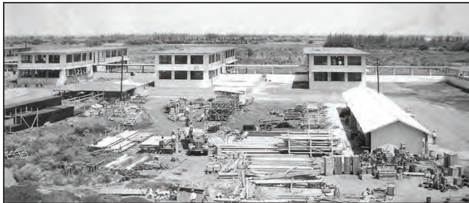
Barracks under construction, August 1940.
