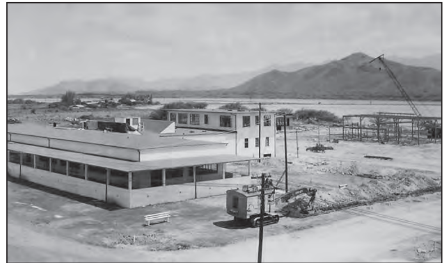
Mess Hall under construction, August 1940.
