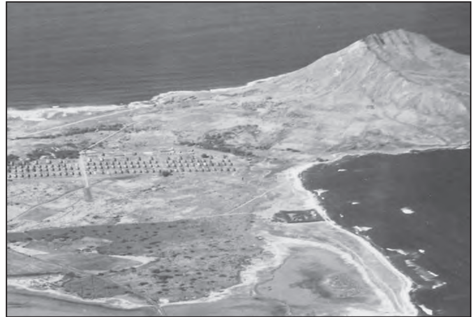
Fort Hase, 1939, view to north.
