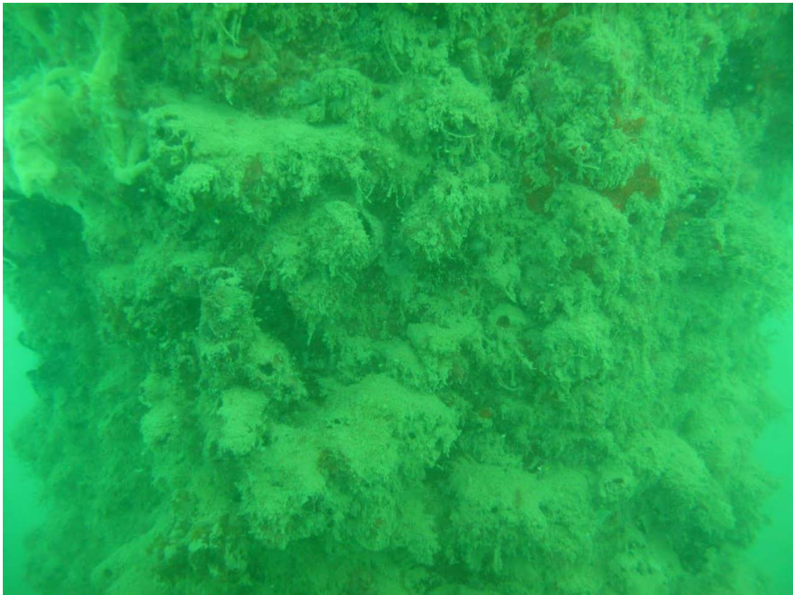
Figure 1 Typical fouling community at a depth of 22 feet.
