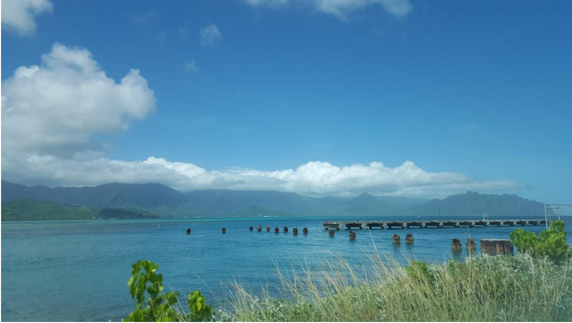
Enclosure 2. Overview of the NOSC pier, view to northwest.
