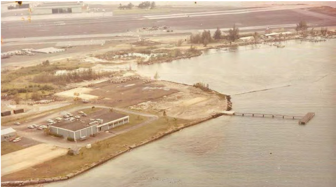
Figure 2. Original configuration of the T-pier, early 1970s
