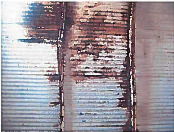
Detail showing rusted framing.
