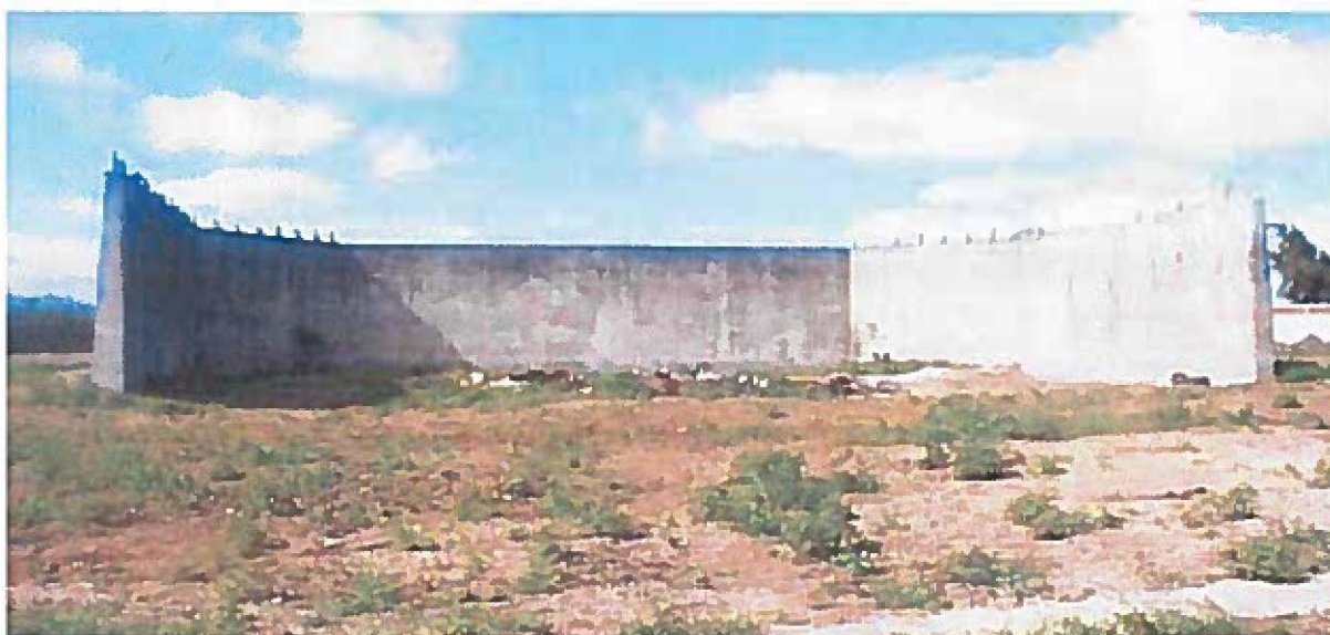
Enclosure 7. Facility 15 showing the steel members that originally held camouflage netting at the top of the wall, view to northwest.
