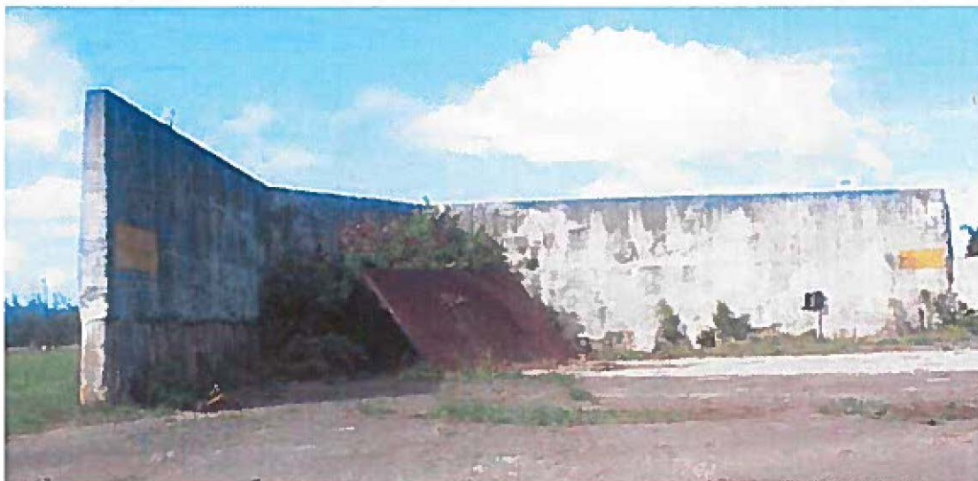
Enclosure 8. Facility 14 with engine check pad inside revetment. Note: the northeastern (right side of image) portion of the wall has been removed, view to north.
