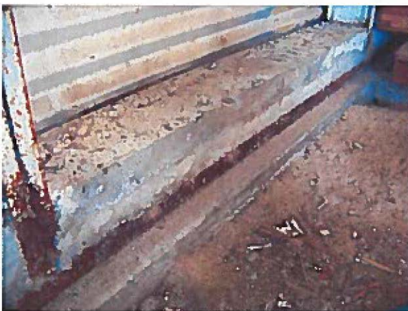
Horizontal ribs embedded in the infill concrete sill.
