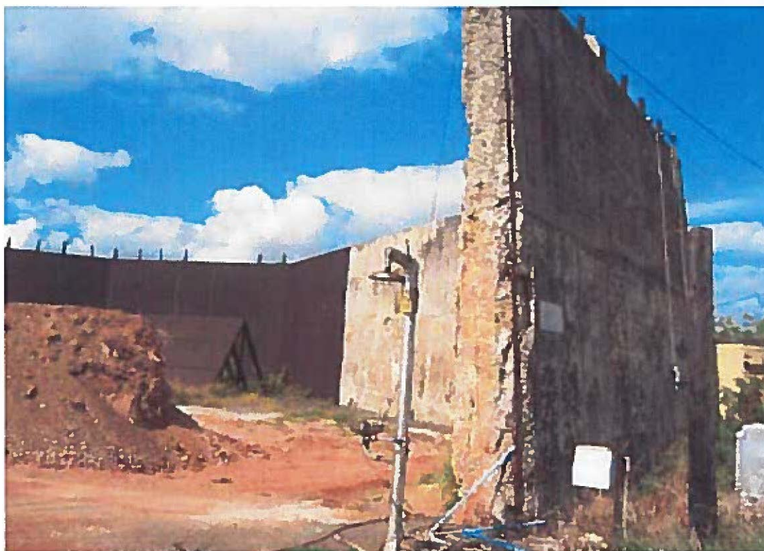
Enclosure 9. Facility 17 showing the engine check pad and steel sheeting in the rear of the revetment. The northernmost wall section (foreground) has been removed. The steel members that originally held camouflage netting are visible on top of the wall, view to southwest.
