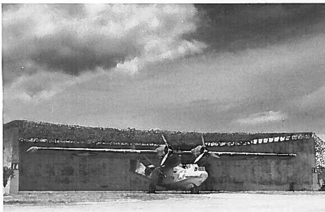
Enclosure 5. Aircraft revetment (Facility 14) at NAS Kaneohe with PBV Catalina. Camouflage netting over the revetment.
