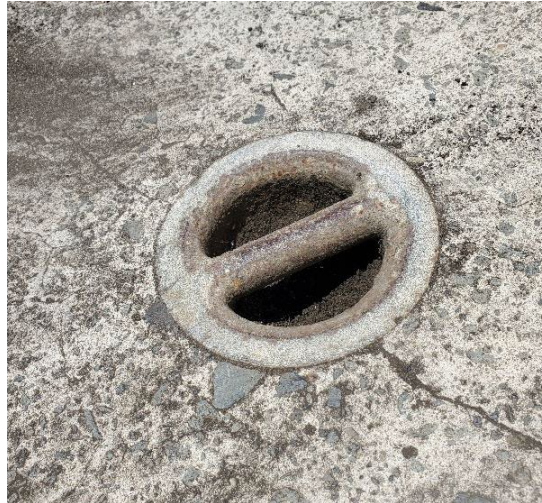
Photo: Example Tie-Down on Bravo Ramp
