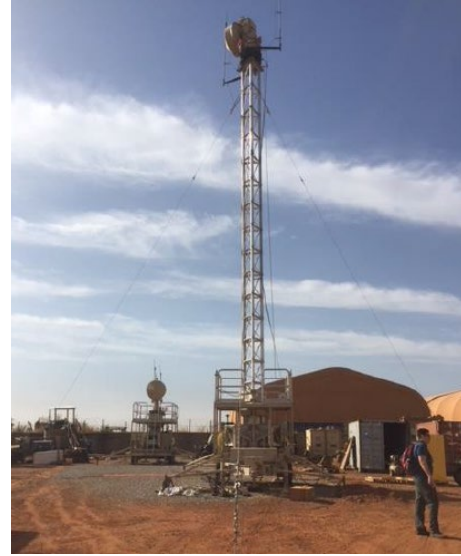
Photo: Representative GDT, Extended with Guy Wires
