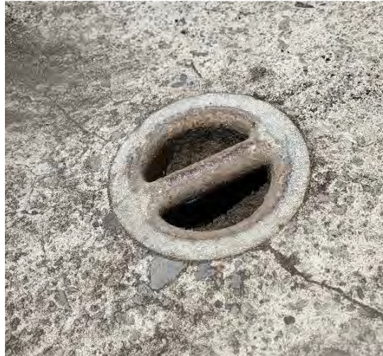
Photo: Example Tie-Down on Bravo Ramp
