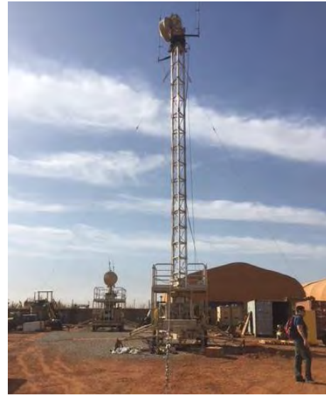
Photo: Representative GDT, Extended with Guy Wires
